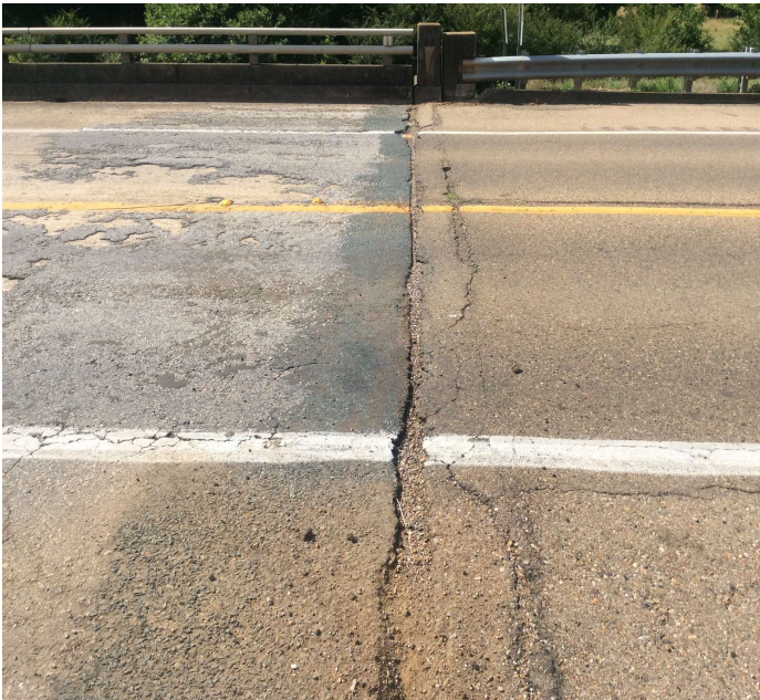
PHOTO 1 Description BEGINNING AND END OF BRIDGE ASPHALT IS BREAKING APART
