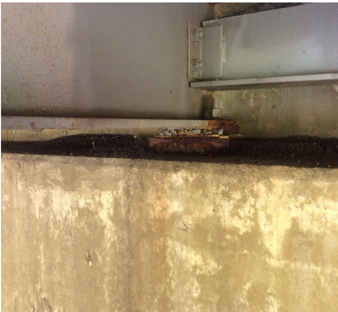
PHOTO 1 Description BEARINGS ARE RUSTING ENTIRE BRIDGE NEEDS TO BE REPAIRED
